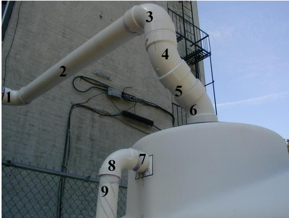
This design uses a separate inflow and overflow pipe.
