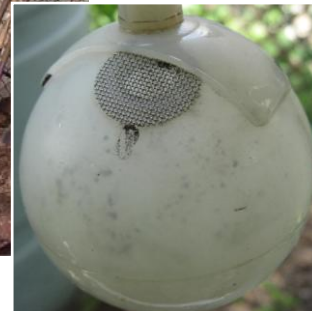
This device allows the overflow pipe to be connected to the roof washer pipe.
